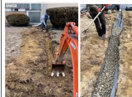
the residence down spout to the parking lot was replaced to prevent water from entering the basement. Pipe was broken during tree work last year. A temporary leader pipe extender was used until repairs were made last week.
